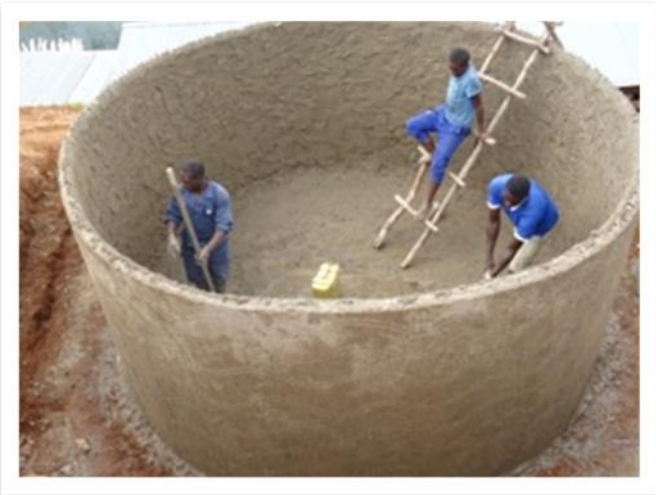
Institution tank (20,000l) constructed by KDWSP masons
