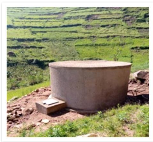
Rainwater tank (4,000 l) constructed by women
